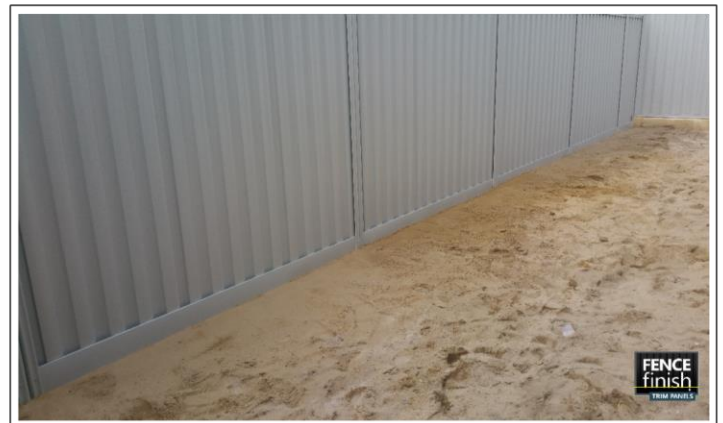
...to an attractive professional finish Fence finished!
